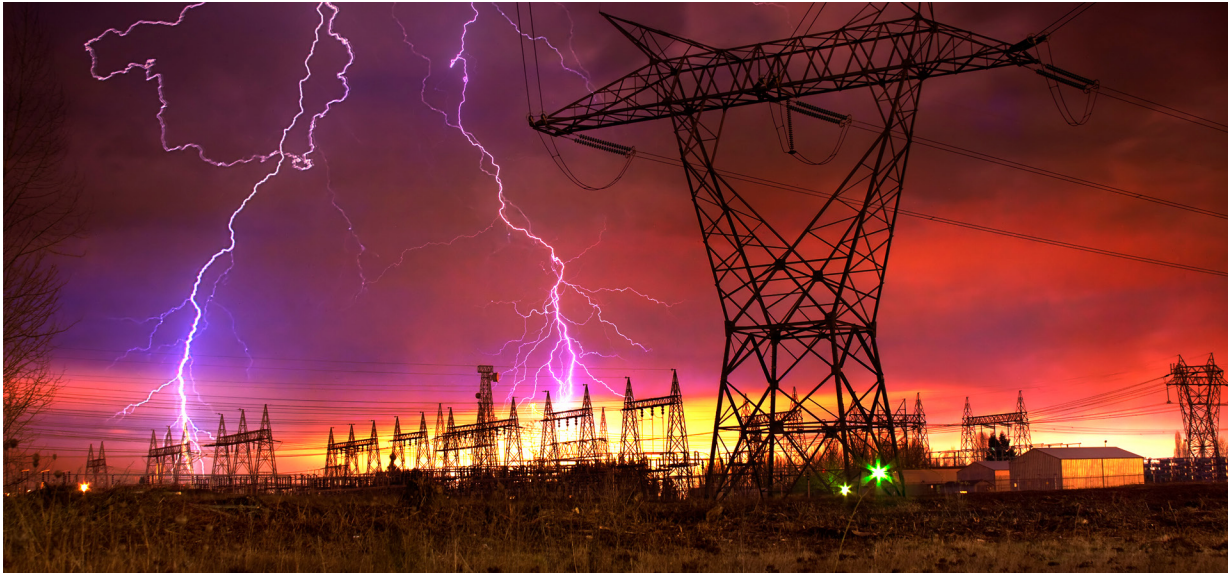
FIGURE 4 – Lightning strike close to an overhead transmission line
